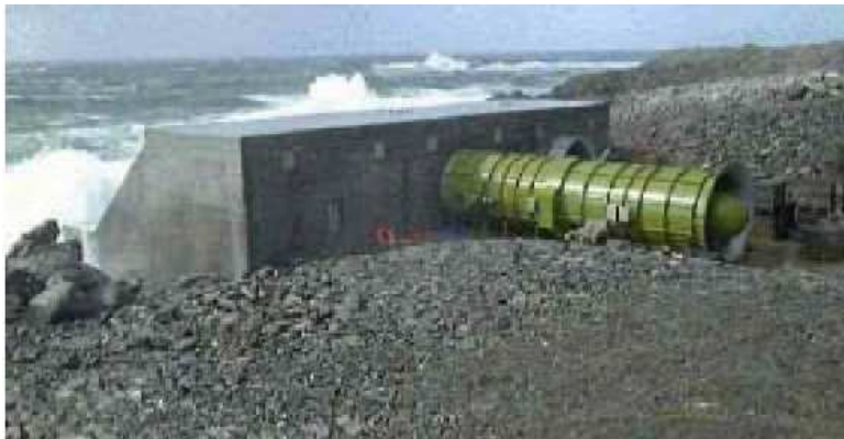
Figure 7: "Limpet" OWC at Isle of Islay, Scotland
