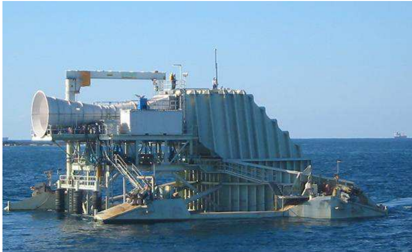
Figure 8: OceanLinx OWC Wave Energy Converter
